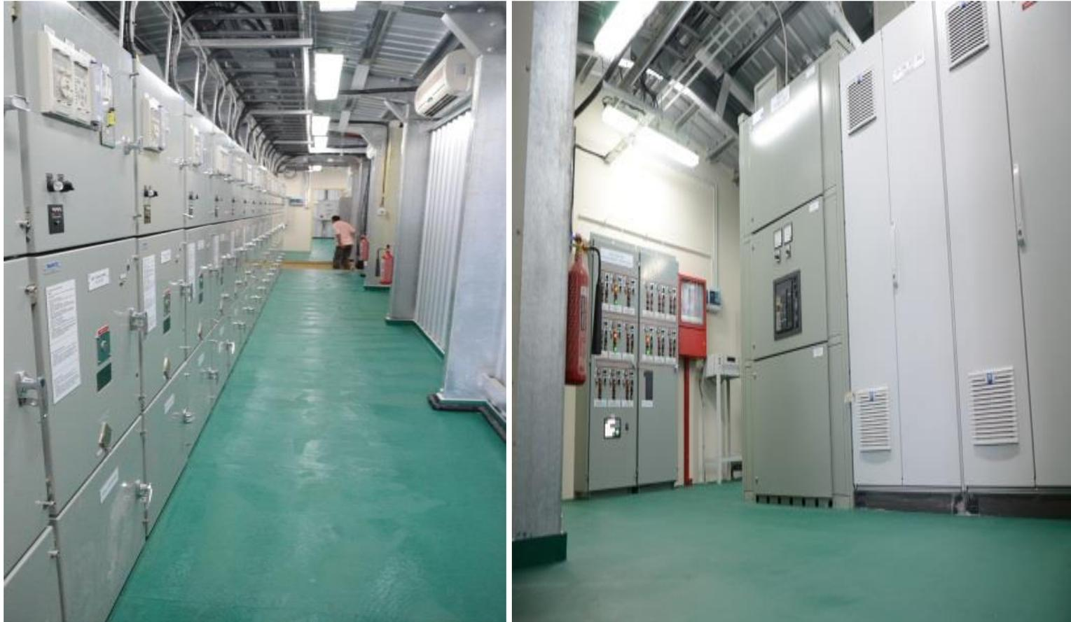
Base frame and steel floor is leveled to switchgear manufacturer's requirement. The floor is installed with fire rated materials to specification.
