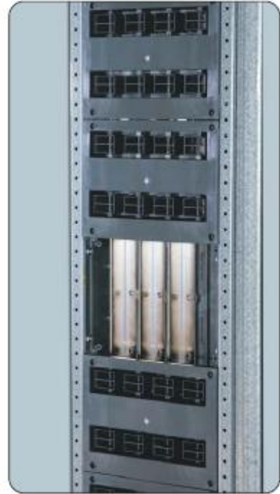
b) Vertical Buses of Withdrawable MCC Cabinet
